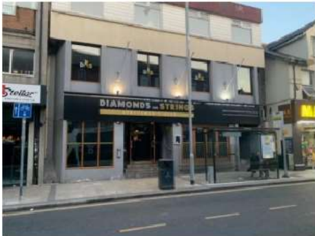
FRONTAGE OF PREMISES DIAMONDS AND STRINGS
